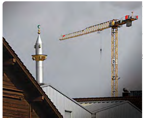
Minaret under construction
