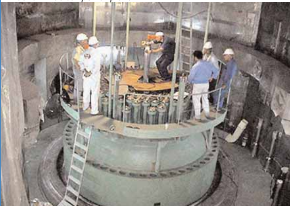
Bushehr nuclear power plant
