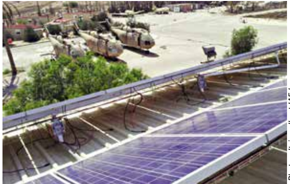
Photovoltaic cells at IAF base
