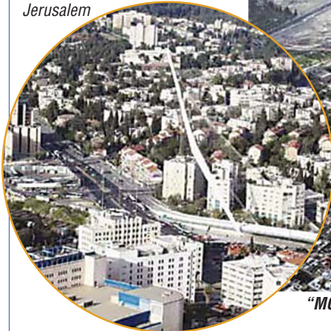
HANGING BRIDGE for the light rail at the entrance to Jerusalem
