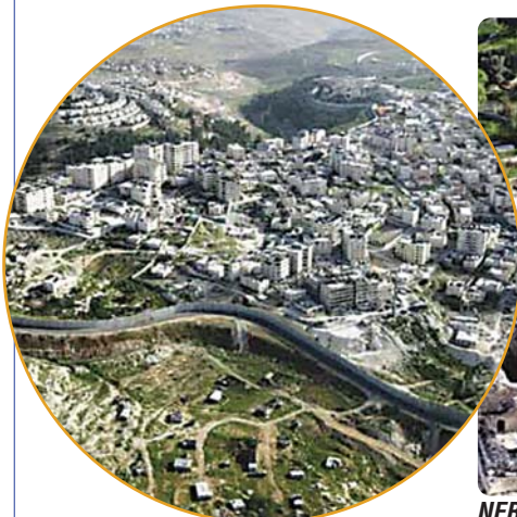
SNAKING BOUNDARY: The security barrier near the Shuafat neighborhood in northern Jerusalem
